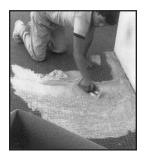
inconsistent application. Consult the adhesive manufacturer for the best application technique. For bonding, the cushion should be laid into the adhesive while in a "tacky wet" condition. For pressure sensitive adhesives,
