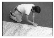
in sufficient amount to achieve full and complete coverage of the cushion and carpet backing, including penetration into the backing's deepest recesses.
