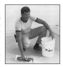
ing to The Carpet & Rug Institute's CRI 104 (2002) Installation Standard, all materials should be acclimated 48 hours prior to installation. If installing over concrete, the slab temperature should not be less than 65 degrees F. The completed installation
