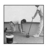
Proper open time considerations are critical for a successful installation. Installing carpet into adhesive without sufficient open time may result in installation failure. The use of fans will reduce the required open time and promote tackiness. However, be aware that excessive moving of the air will accelerate the drying time and may not achieve a transfer of adhesive to the backing of the carpet.
