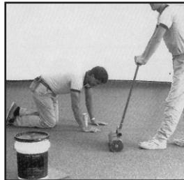
Prevent all traffic over carpeted area for a minimum of 24-48 hours after installation. Failure to do so may create areas where inadequate adhesion between carpet and cushion can lead to future performance problems.
