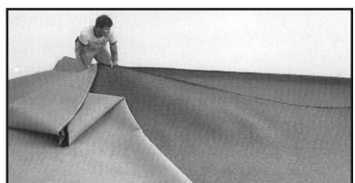
Once the entire cushion has been laid out, fold it back and apply adhesive to the floor. Do not staple. Direct special attention to spreading the adhesive adjacent to the walls (cut-in) to prevent edge curling. Apply the adhesive with a u-notched trowel measuring 1/16 x 1/16 x 1/16 inches, or according to the adhesive manufacturer recommendations. Applying the adhesive with a paint roller can result in an inconsistent application.
