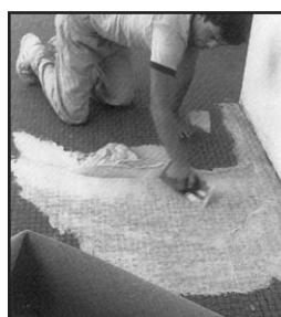
Consult the adhesive manufacturer for the best application technique. For bonding, the cushion should be laid into the adhesive while in a "tacky wet" condition. For pressure sensitive adhesives, this point is often identified when the adhesive turns clear from its original opaque appearance. Smooth the cushion into the adhesive, working toward the seams. Trim in, eliminating any bubbles or wrinkles so that the seams are tight without overlapping.
